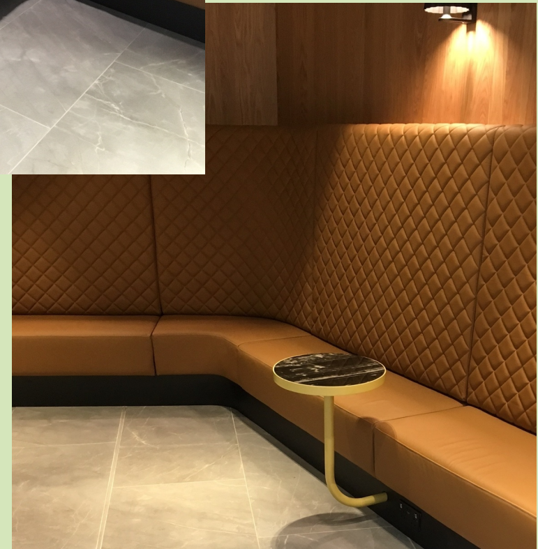
- Walnut veneered wall panels set into an anodise aluminium extrusion.
